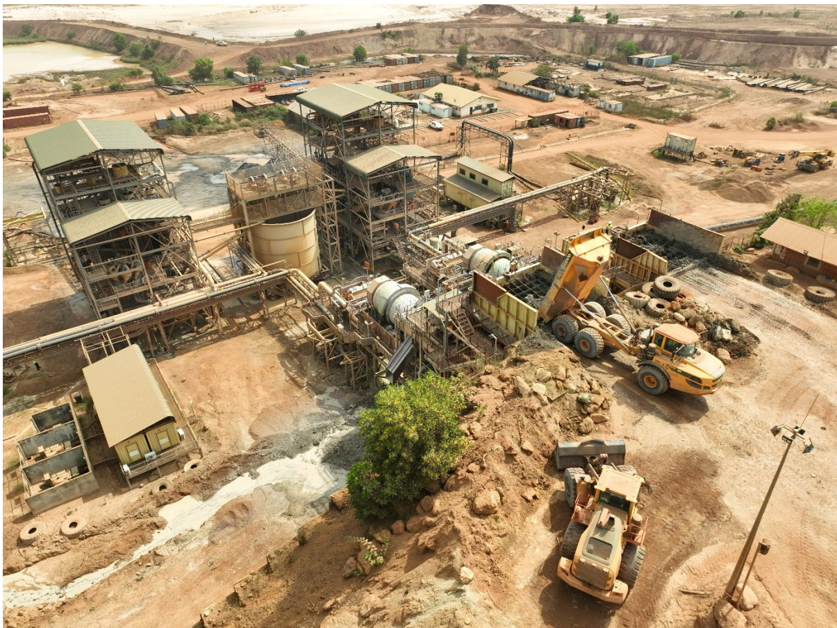
Aerial view of DM2 WMC at Gangama
